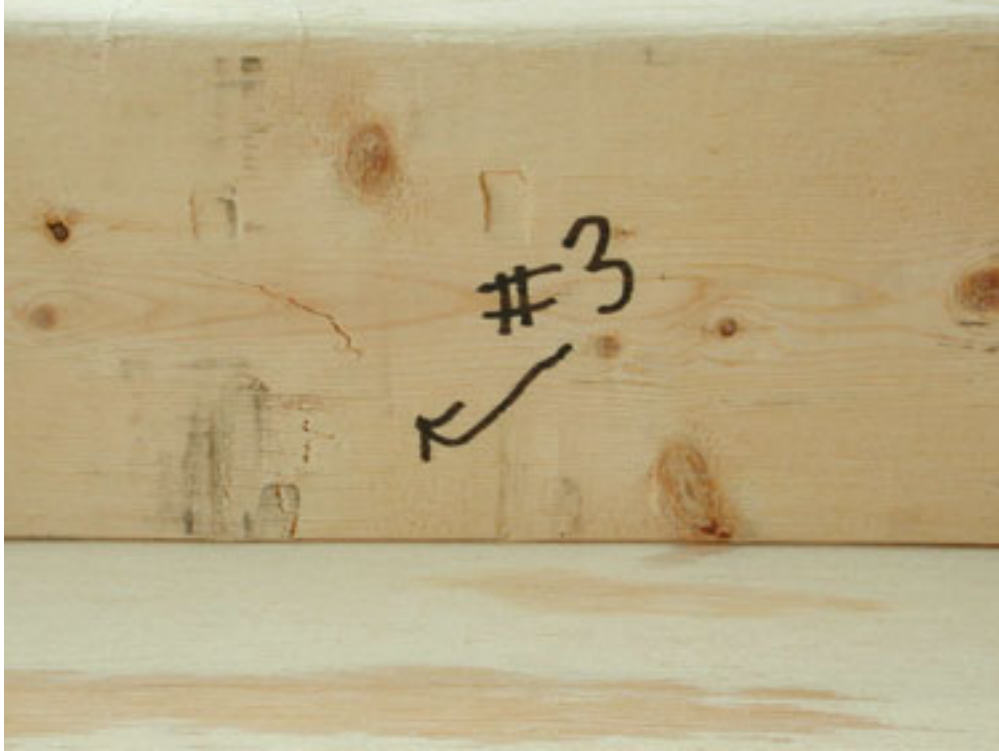
PHOTOGRAPH 25 SPECIMEN 3 FAILURE OF 2 x 4 STUD
