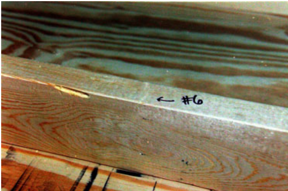
PHOTOGRAPH 32 SPECIMEN 6 FAILURE AT 2 x 4 STUD
