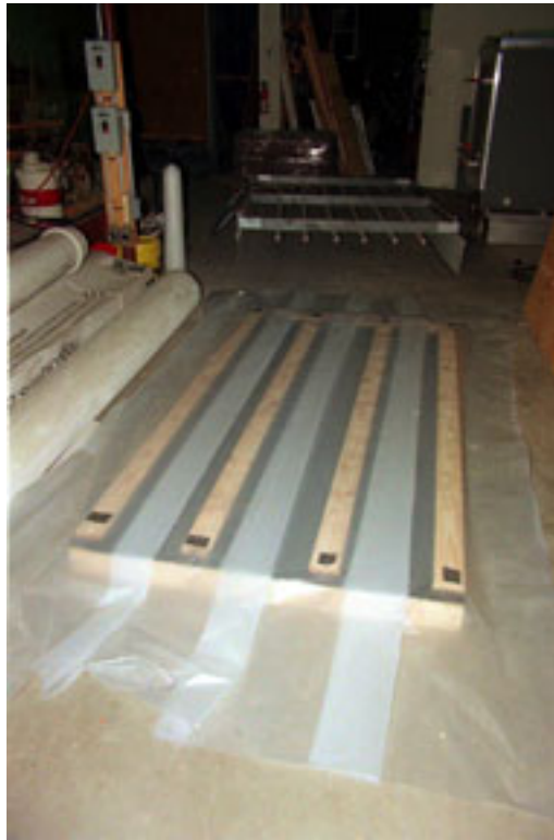
PHOTOGRAPH 13 POLYETHYLENE SHEET ATTACHED TO FRAME
