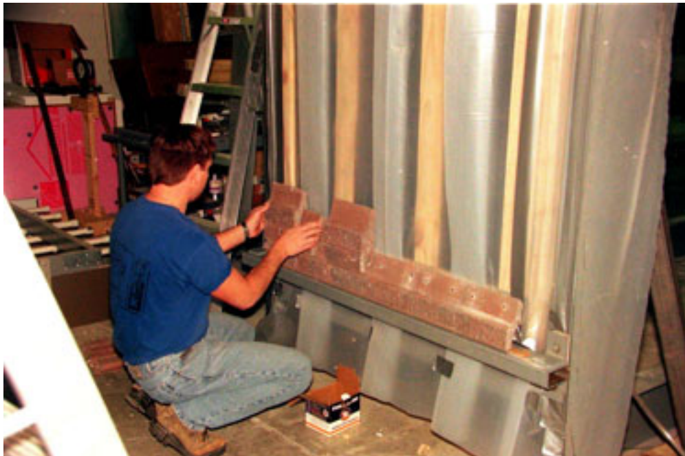
PHOTOGRAPH 16 RUNNING BOND PATTERN ASSEMBLY OF NOVA BRIK PANEL
