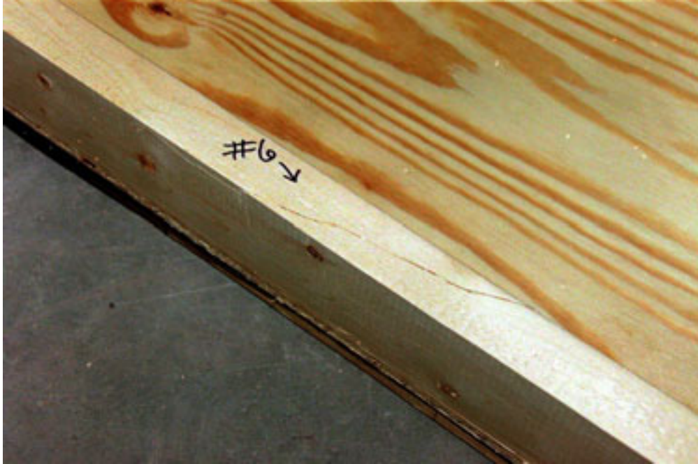
PHOTOGRAPH 31 SPECIMEN 6 FAILURE AT 2 x 4 STUD
