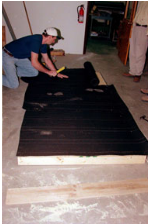
PHOTOGRAPH 11 ATTACHMENT OF FELT PAPER TO FRAME
