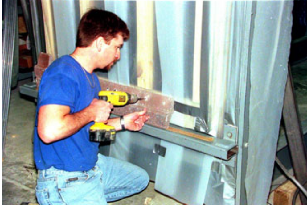
PHOTOGRAPH 15 ATTACHING THE FIRST COURSE TO THE BASEBOARD
