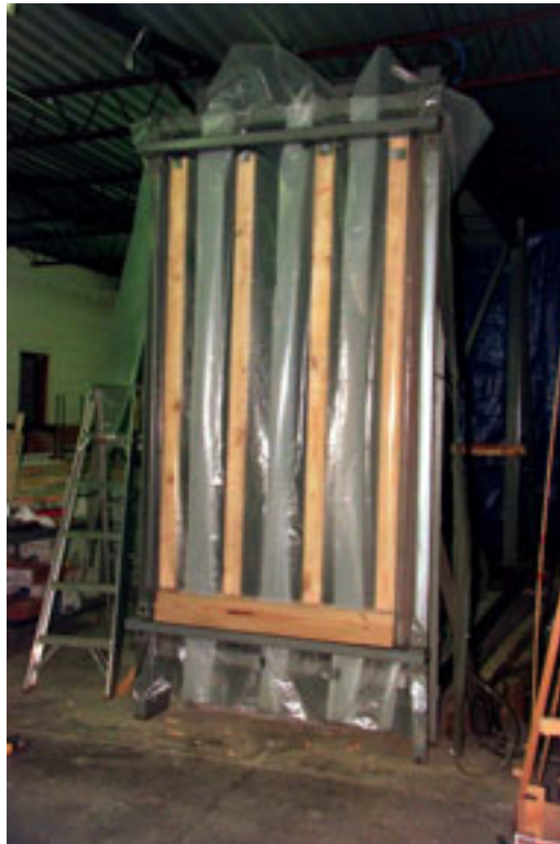
PHOTOGRAPH 14 FRAME IN PLACE IN TEST CHAMBER; READY FOR NOVA BRIK
