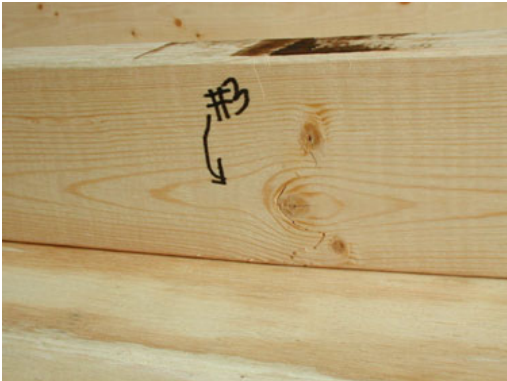
PHOTOGRAPH 24 SPECIMEN 3 FAILURE OF 2 x 4 STUD
