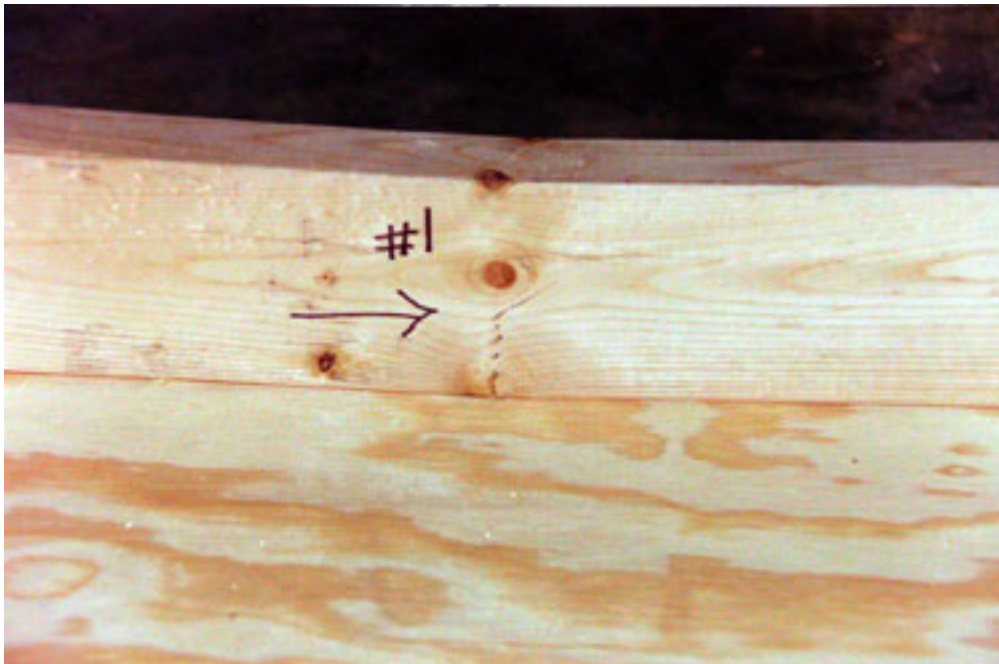
PHOTOGRAPH 20 SPECIMEN 1 FAILURE OF 2 x 4 STUD
