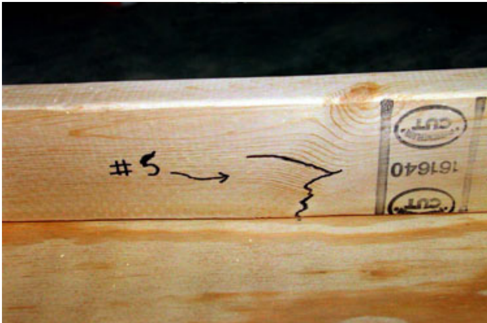
PHOTOGRAPH 30 SPECIMEN 5 FAILURE OF 2 x 4 STUD
