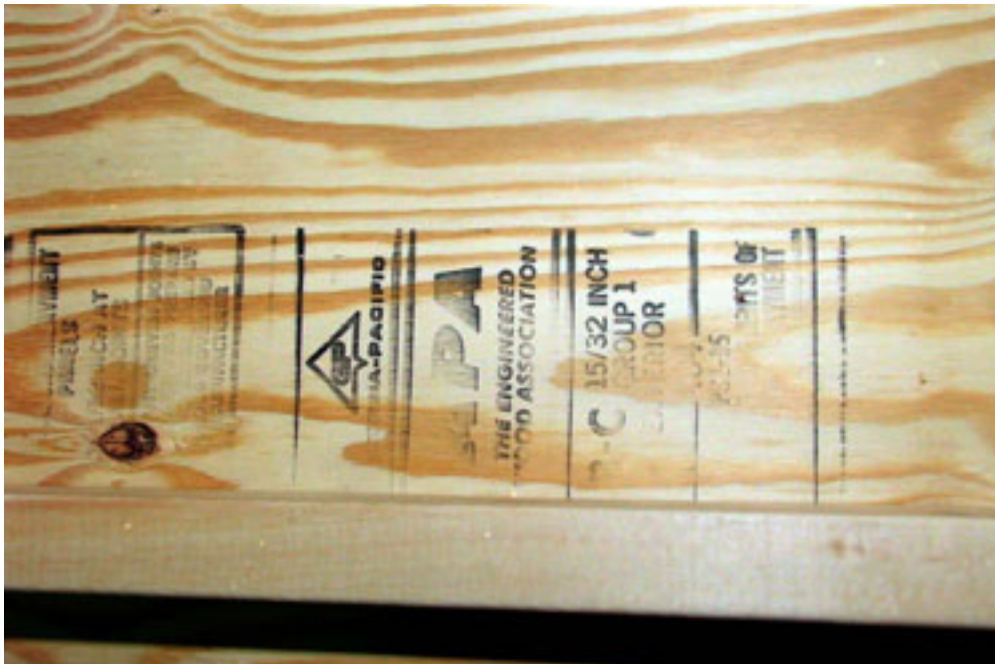
PHOTOGRAPH 10 BC GRADE PLYWOOD USED ON SUPPORT FRAMES
