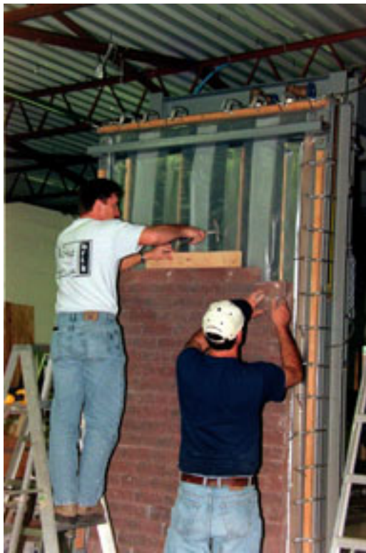
PHOTOGRAPH 17 CONSTRUCTION OF NOVA BRIK WALL PANEL
